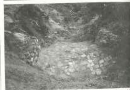
A weir constructed with effective involvement of people holds water (photo 1), while another weir lower down constructed earlier was always dry (photo 2). Note the wall protecting a large area in photo 1.
