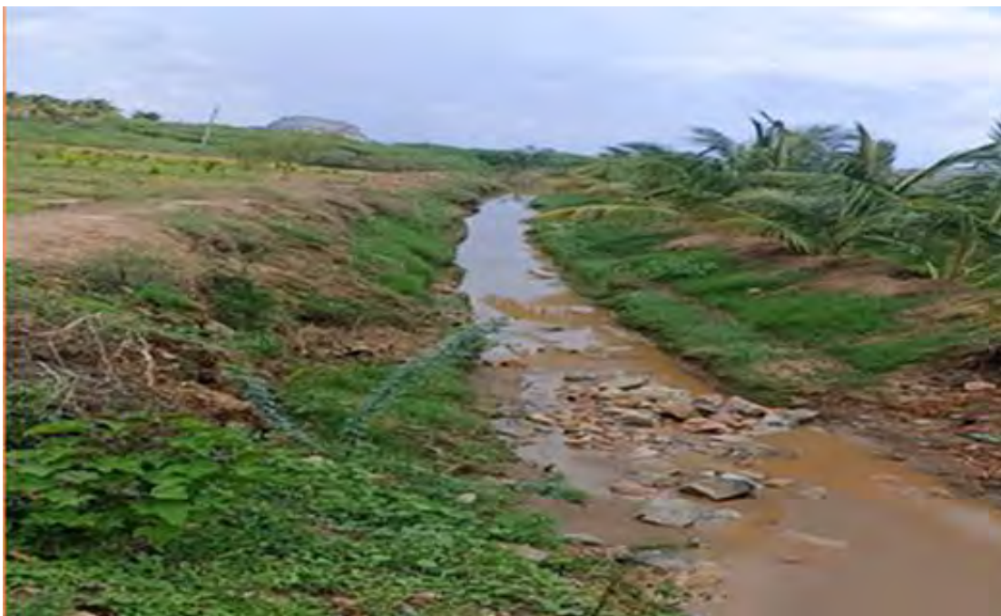
Photos: Newly constructed feeder channel guiding surplus runoff from agricultural fields into the tank system, preventing erosion and restoring natural inflow patterns.
