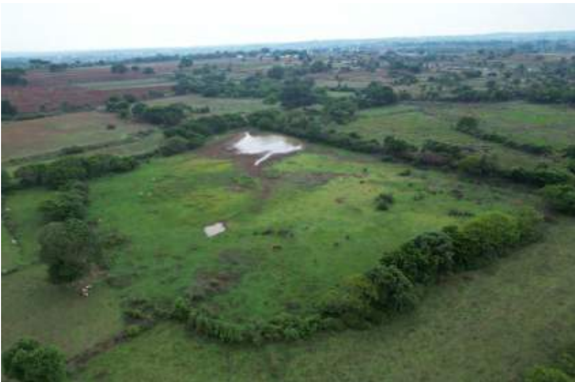
Photo: Severely silted irrigation tank with limited water storage capacity, highlighting reduced holding potential and declining reliability for agriculture.
