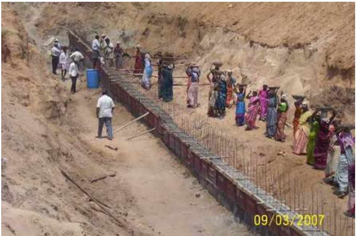
Photos: Construction of a subsurface dam below ground level using earth-moving equipment and manual labour, capturing the landscape context and scale of intervention.
