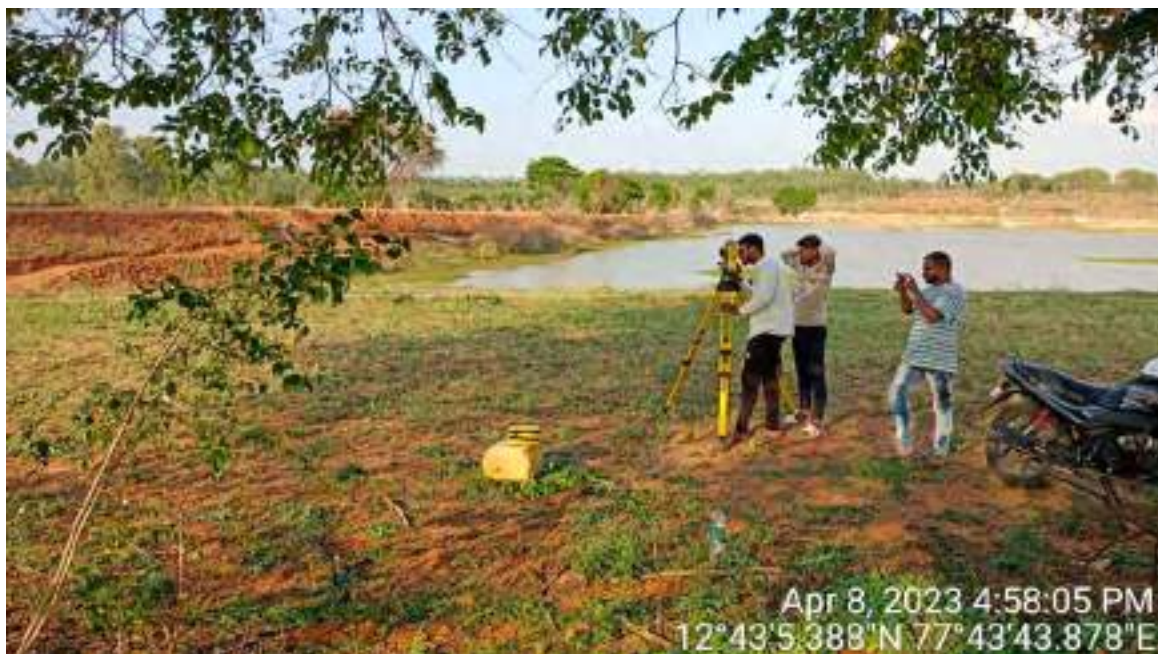
Photo : Technical assessment using Total Station survey to estimate silt volume, map tank contours, and plan systematic desilting and storage enhancement.
