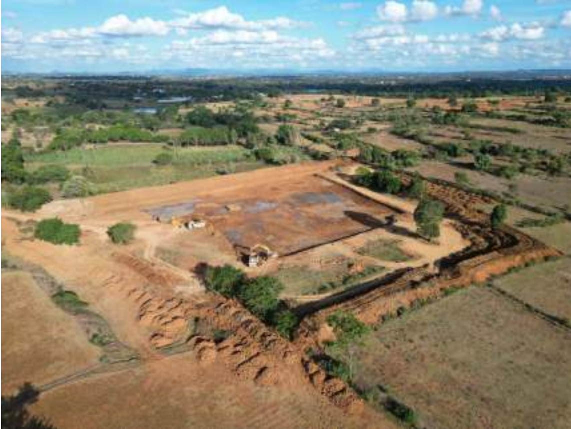
Photo: Tank desilting in progress with removed silt and strengthened bunds, restoring storage capacity and improving structural stability.
