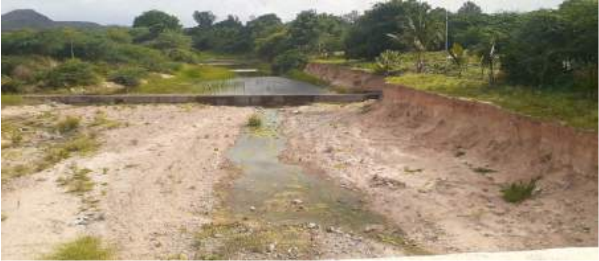
Photo: Completed subsurface dam with only a low masonry section visible above ground, illustrating how water is stored within the soil profile with minimal surface storage.
