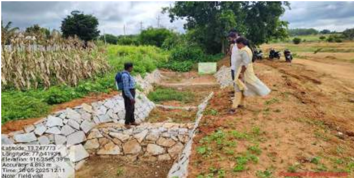
Photo: Completed drainage line treatment with loose boulder checks, grass filters, and sand filter chambers, demonstrating on-ground implementation of decentralised wastewater treatment and improved water quality.
