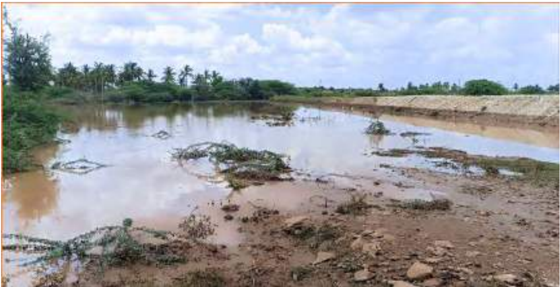
Photos: Strengthened and widened tank bund to enhance storage capacity and safety during high inflow
