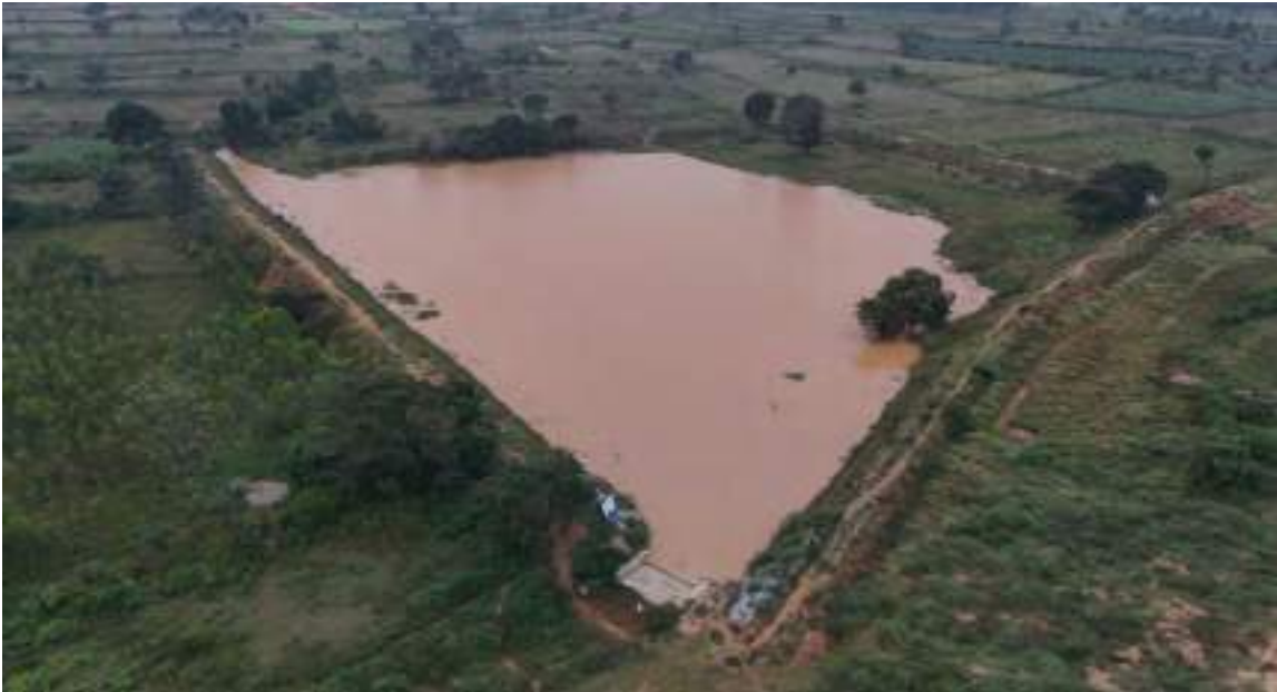
Photo: Revived tank with increased water storage and improved surplus weir height, ensuring enhanced water availability and safe overflow management.
