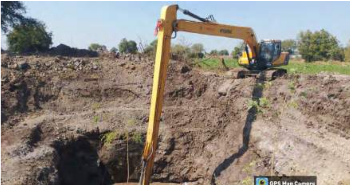
Photo: Long-reach excavator used for efficient desilting and deepening of an open well
